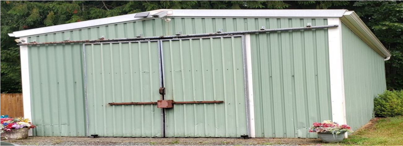
Maintenance shed where we would like power for lights & security
